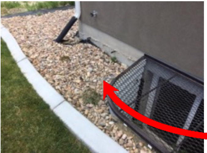
Rear Exterior Landscaping Settling
