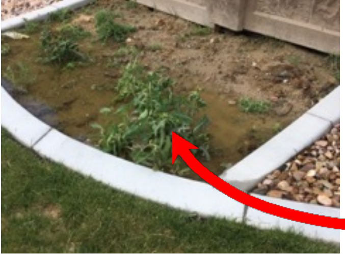
Rear Exterior Landscaping Potential drainage issue
