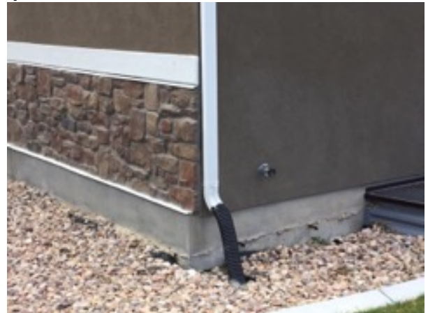
Downspout/ Splash Blocks
