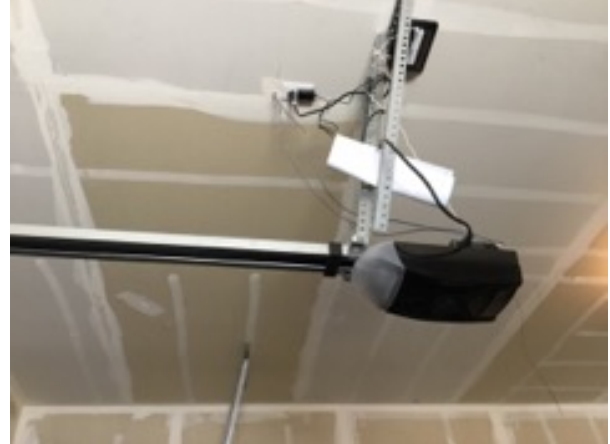
Garage Door Electric Opener
