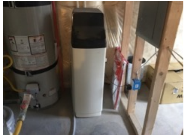
Water Softener System
