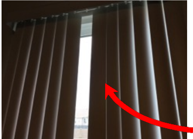
Blinds/Drapes - Missing vane
