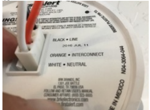
Smoke Alarm (DATE)
