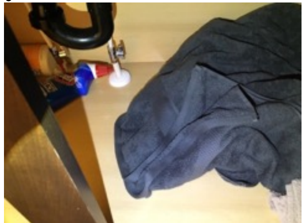
Cabinet Under Sink
