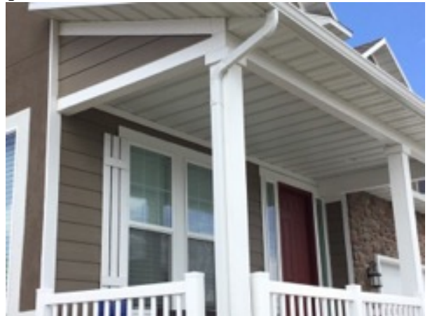
Downspout/ Splash Blocks
