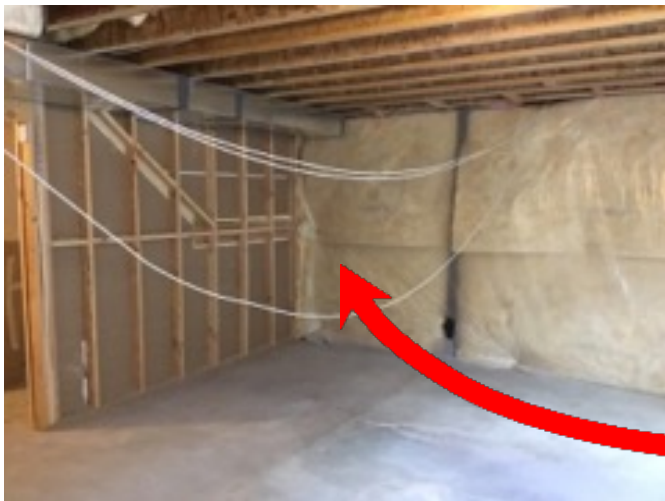
Basement Overview Wires hanging down
