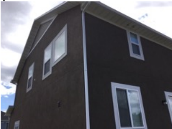
Downspout/ Splash Blocks
