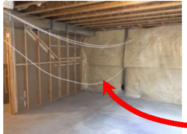
Overview - Wires hanging down
