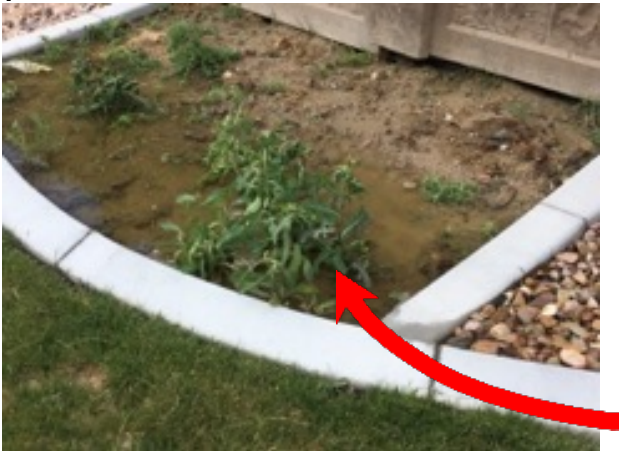
Landscaping - Potential drainage issue
