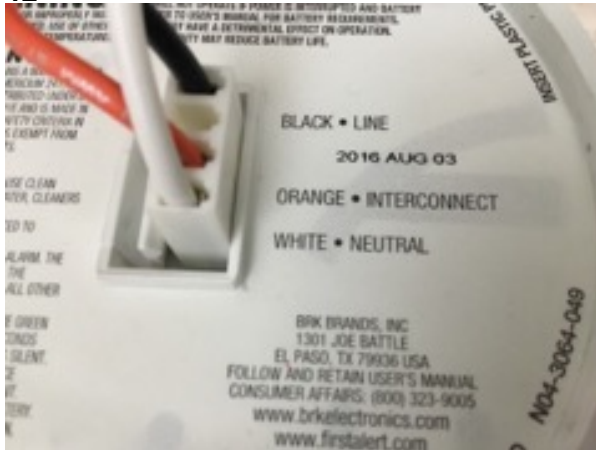
Smoke Alarm (DATE)
