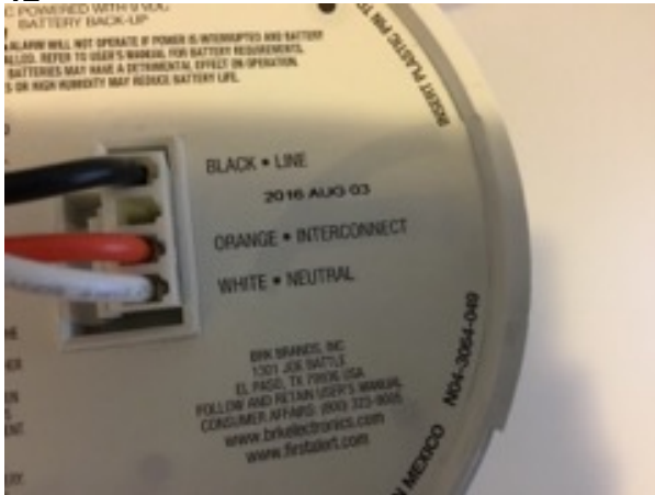
Smoke Alarm (DATE)
