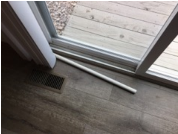
Sliding Door Secondary Lock
