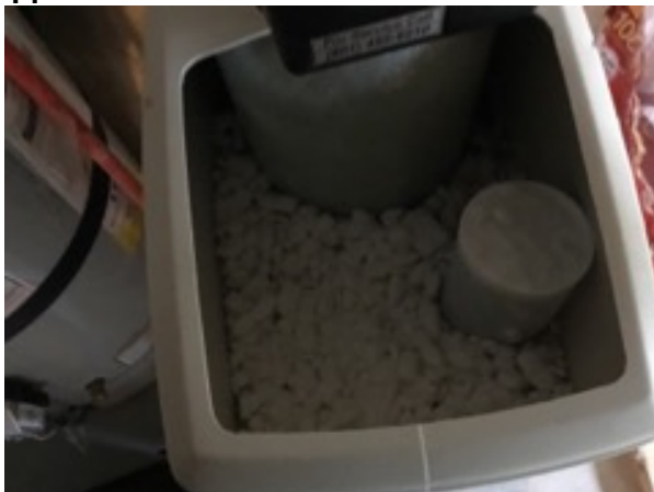
Interior of Brine Tank
