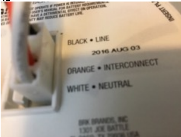
Smoke Alarm (DATE)
