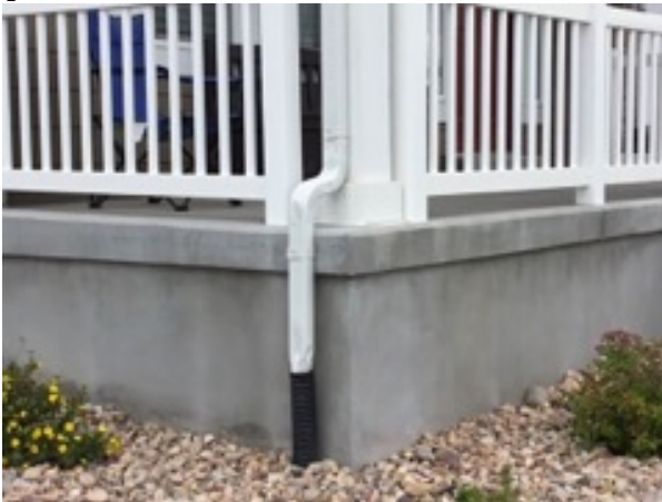
Downspout/ Splash Blocks
